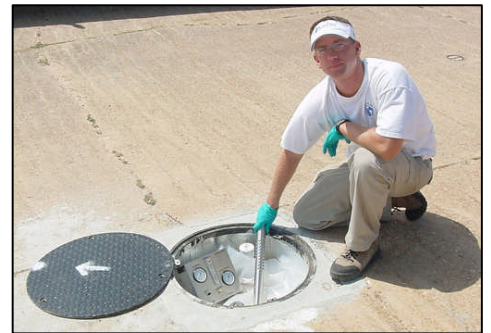
Figure 2: Installation of the iSOC™ and oxygen tank in well vault.
